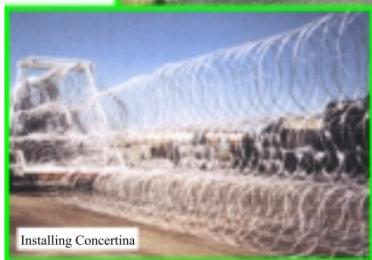
Enhanced Border Barrier with 6 Rolls of Concertina
